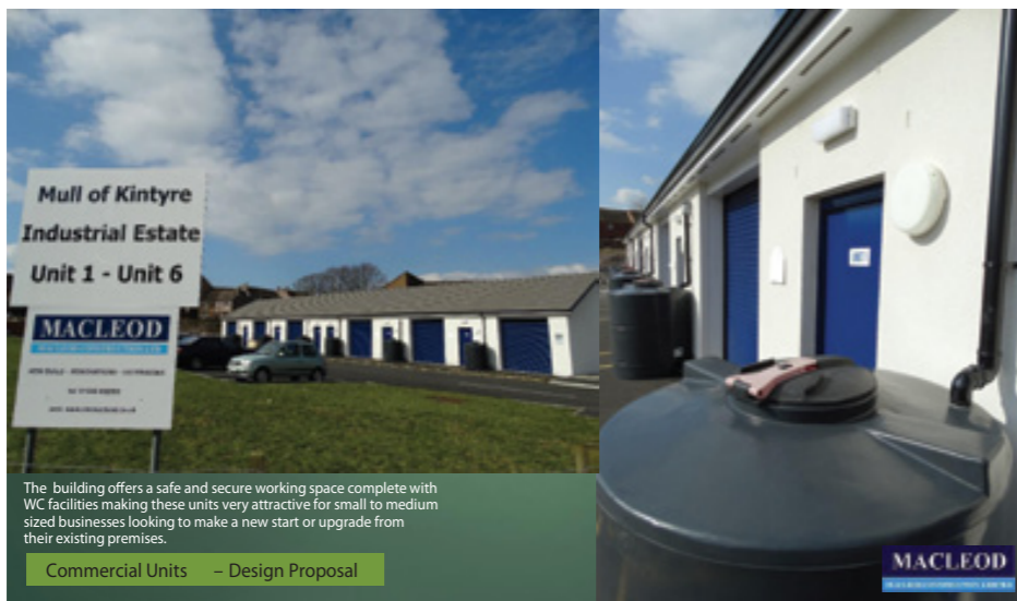
MacLeod Construction workshops at Campbeltown
